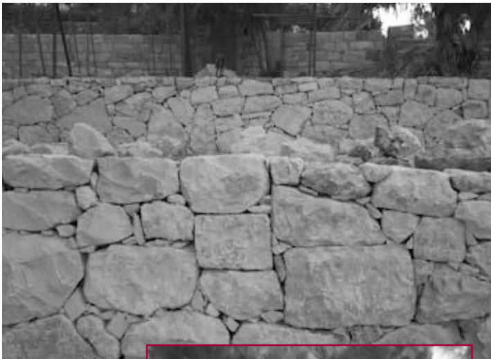
Above: A retaining wall, sanasel , is a structure that holds soil or rock from a building area. It also prevents down slope movement or erosion and provides support for vertical or near-vertical grade changes.
