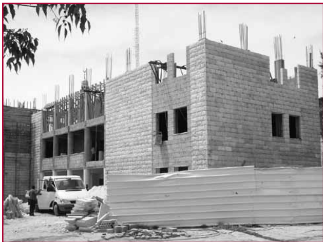
New classroom building is nearing completion
